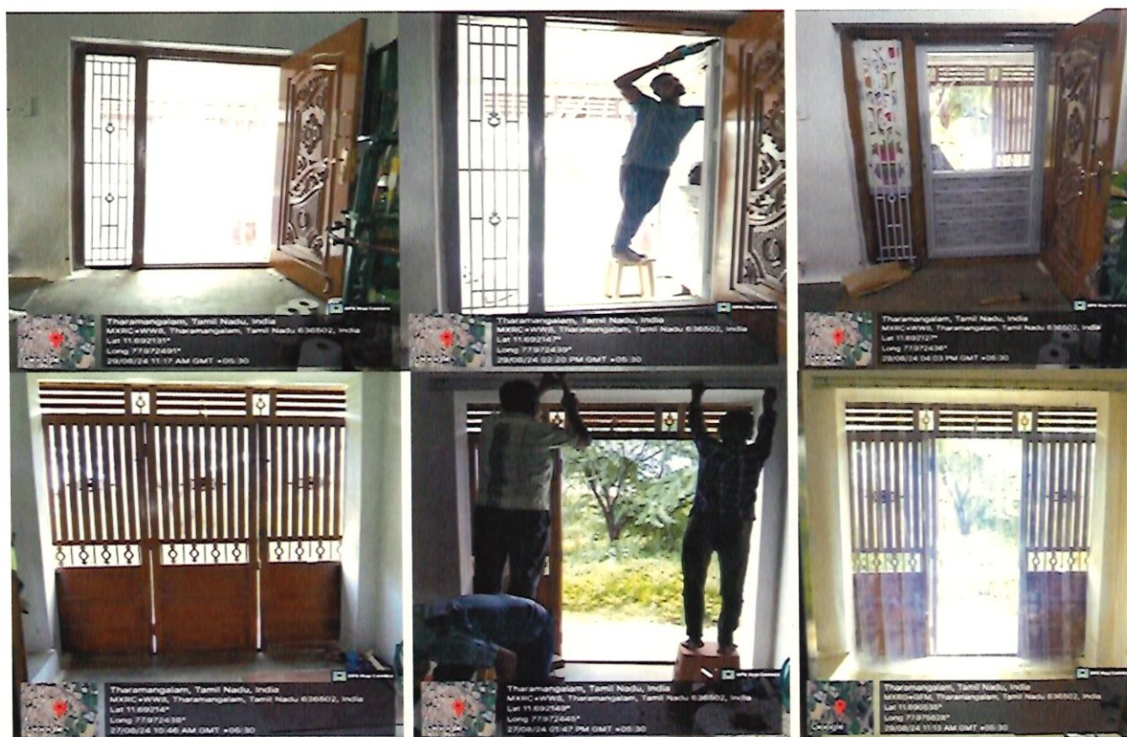
Figure 4.14: Installation of control measures at Transmission path
